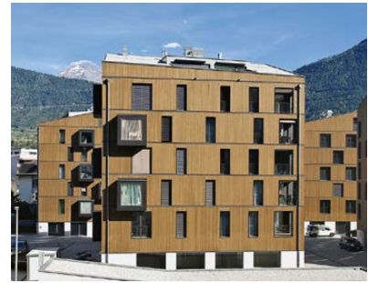
Aletsch Campus in Holzmodulbauweise.
